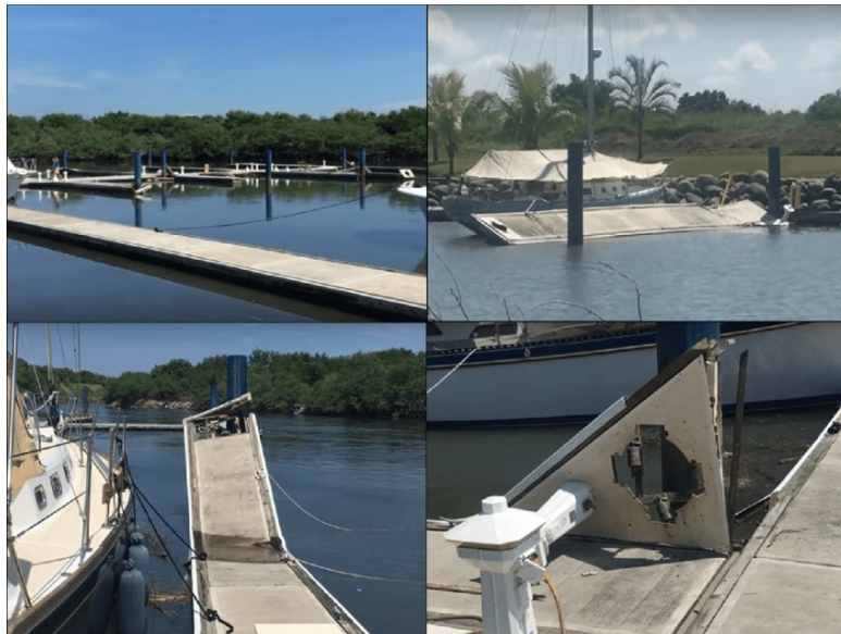
Figure 41: Dock damage in Marina Chiapas after the 2017 earthquake and tsunami. (María Teresa Ramirez-Herrera, 2017)
