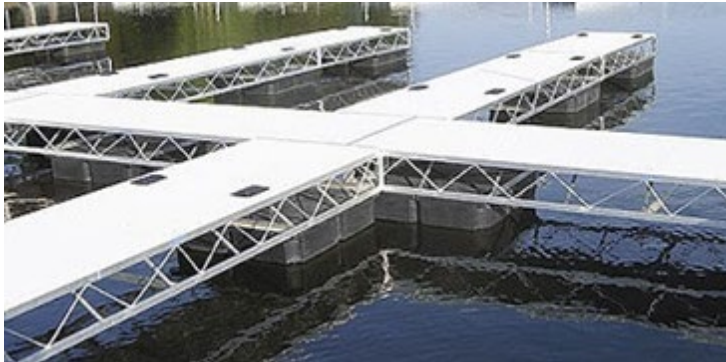
Figure 44: Docks on floating Styrofoam blocks.
