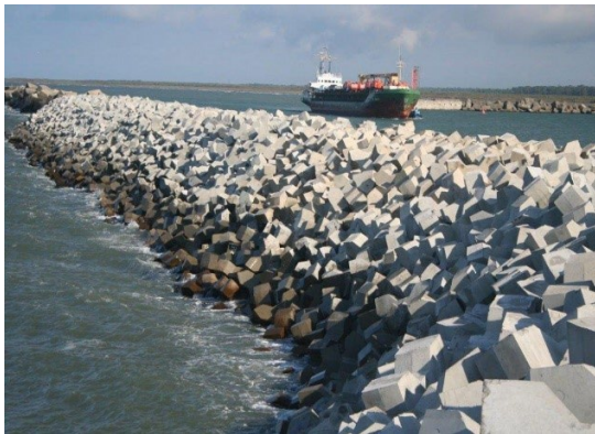
Figure 50: Photo of fortified breakwater off marina.
