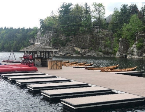
Figure 45: Docks built on full floatation.
